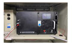
The transformer is a ferro-resonant constant voltage transformer which ensures a clean power output. With the Inverter module, the interface to the whole power system is accomplished through a color touchscreen display for setup, control and monitoring of the system. An optional status monitoring module is available with a DOCSIS Modem for remote monitoring.
